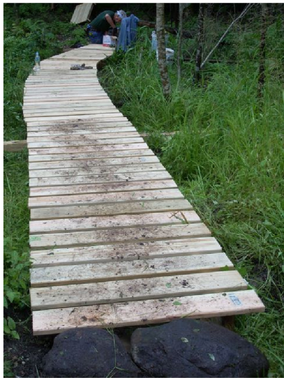
Bridge near West Road. It is located near a rustic cedar bench.
