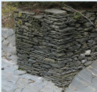
◀ **FLOODING** | Flooding took out the Boston-Albany Post Road bridge that used to span the river here. But the old bridge abutment, built about 1764 using a schist called Goshen stone, has lasted well.
